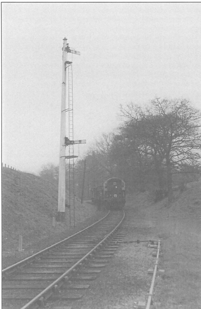
Fig. 42 Class 15 approaching the junction. Notice how the top home signal is set obliquely to the line so that it can be clearly read further down the line and round the curve. Dr. Allen.
