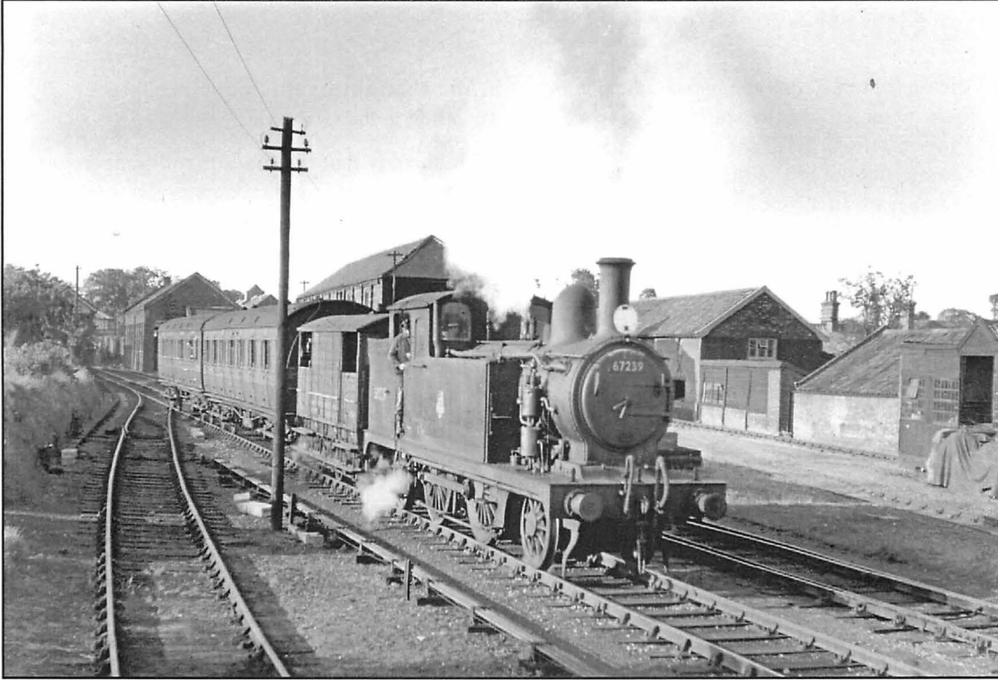
Fig. 17 F6, 2-4-2, number 67239, showing the Westinghouse brake system, hauling the normal branch passenger train out of Framlingham, unusually front first. Dr. Allen
